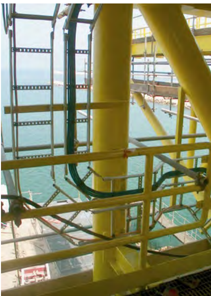
Wibe KHZP tikashylyy asennettuna BP/ARCO/Technip – Al Rayyan Development, Qatar.
